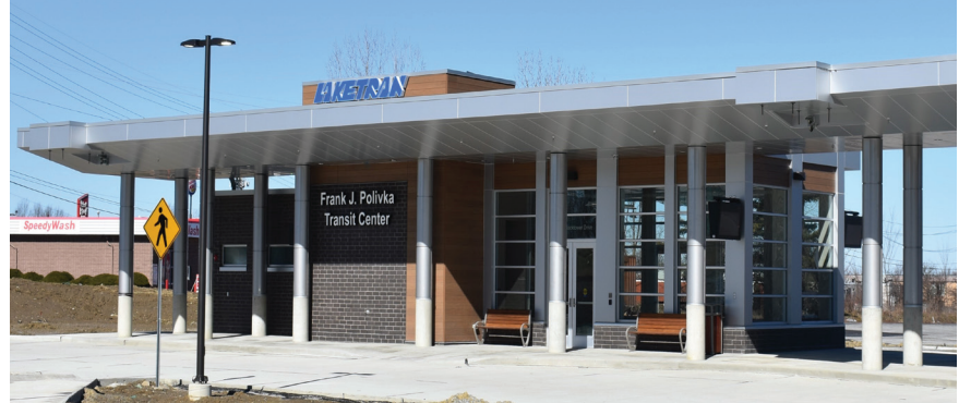
Laketran's new Frank J. Polivka Transit Center at Lakeland Community College includes charging infrastructure—ready to deploy the agency's first battery-electric buses this summer.
